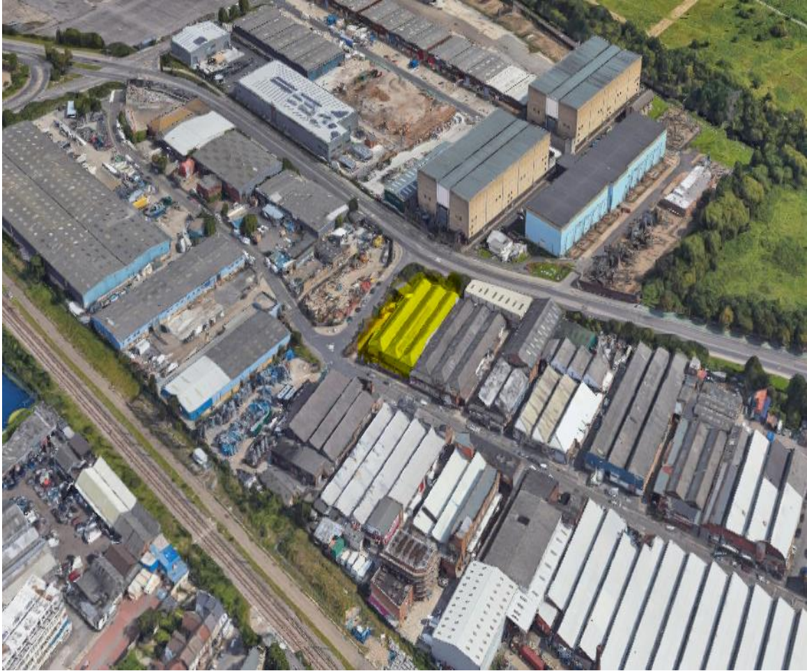
Image 2 Aerial view of the site
