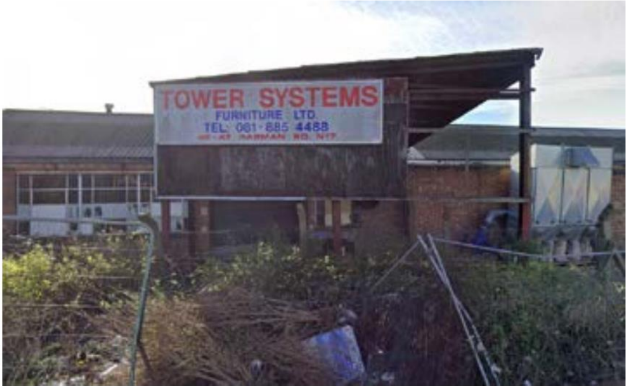
View from roundabout on north-west corner
